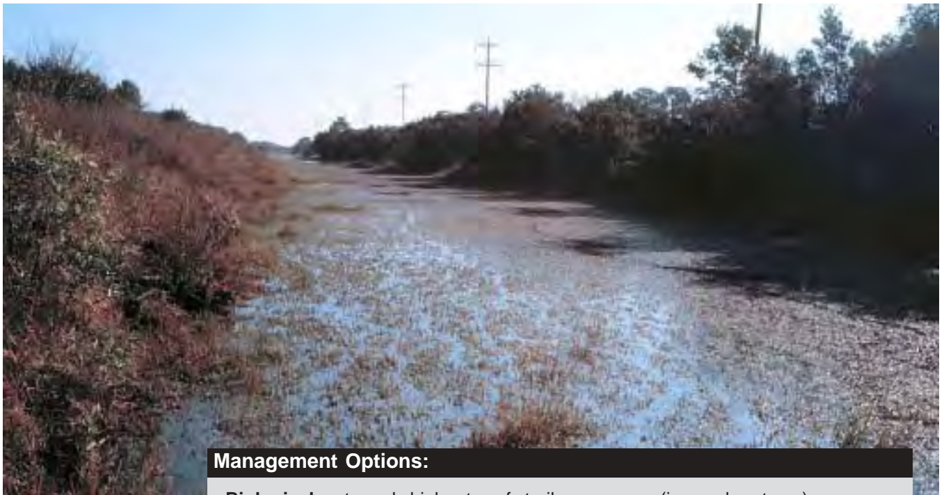
Hygrophila clogging a South Florida flood control canal
