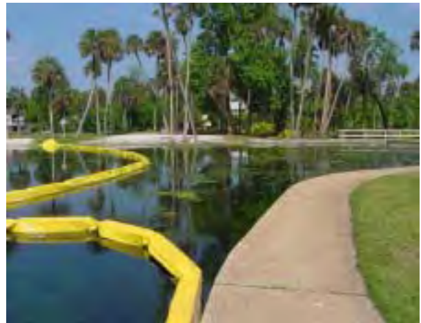
Applying endothall herbicide behind silt barrier in Sanlando Springs (above)
