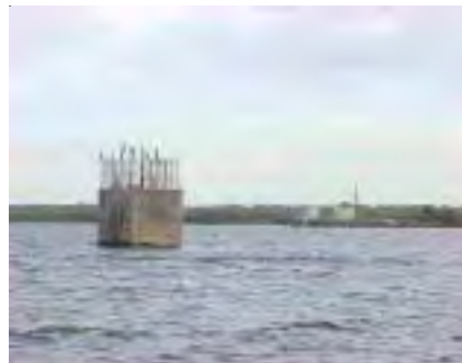
Potable water intakes on lake Washington
