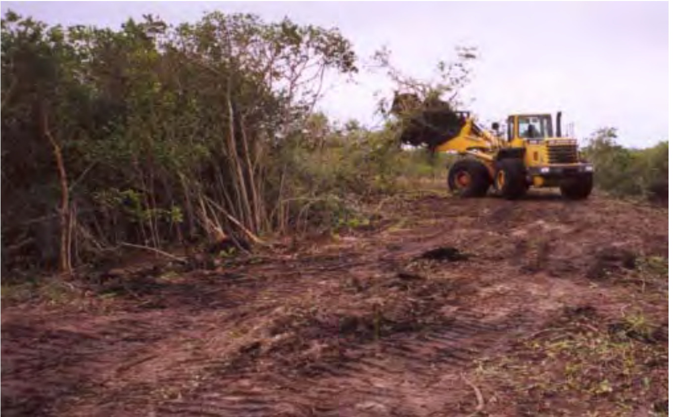
The heavy equipment rolls in...
