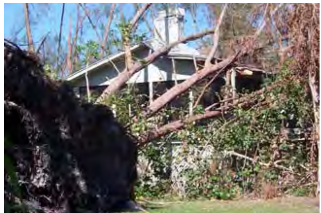
The shallow root system of the Australian pine makes the tree susceptible to “tipping.”
